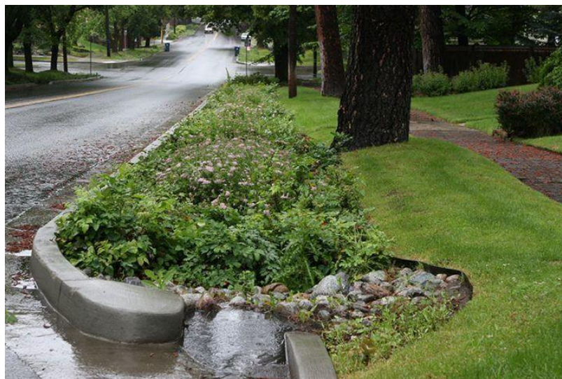
Figure 6: Example of Curbside Rain Garden in Residential Area
