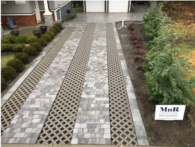
Above: Example of on-site pervious paving Photo Credit: mnrhardscaping.ca
