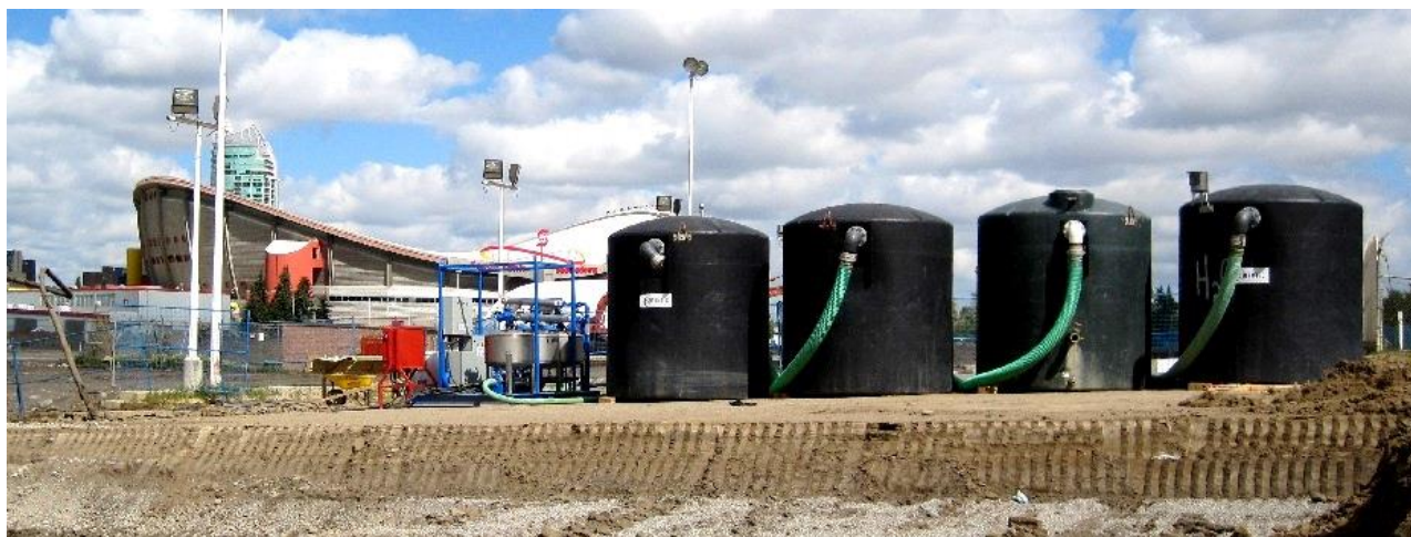
Figure 15: Example of sediment-laden water storage tanks (photo source Stormtec)
