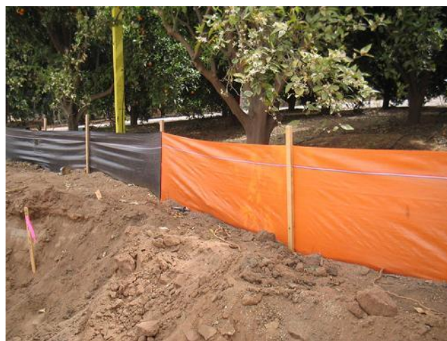
Figure 14: Silt Fence and Posts (photo source BMP Supplies)
