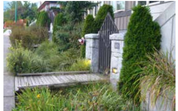
Boardwalk Crossing Over Bioswale
