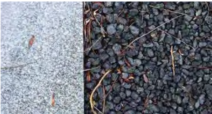
Stone paving by aggregate paving
