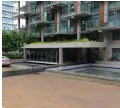
Avoid Wide Expanses of Hard Surfaces in Front of Buildings
