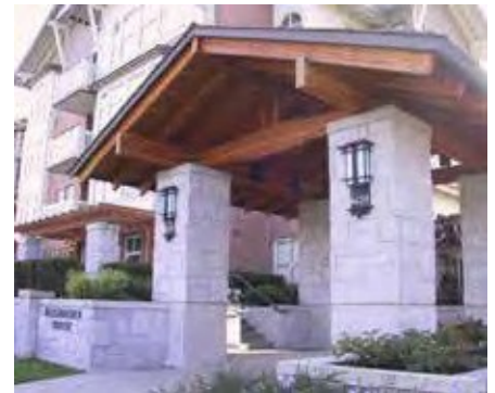
Highly Visible Lobby Entry
