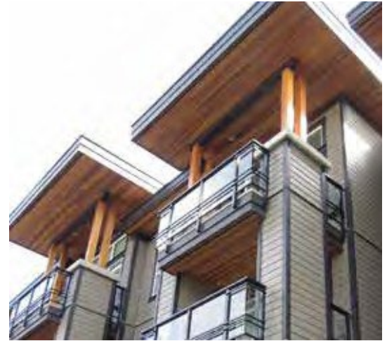
Cedar Soffits Protected from Weather
