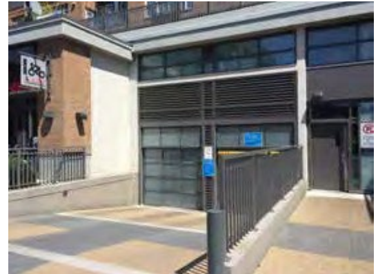
Loading Bay with Doors
