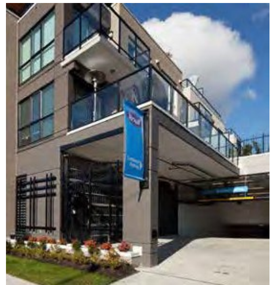
Garbage and Recycling Enclosed within a Building
