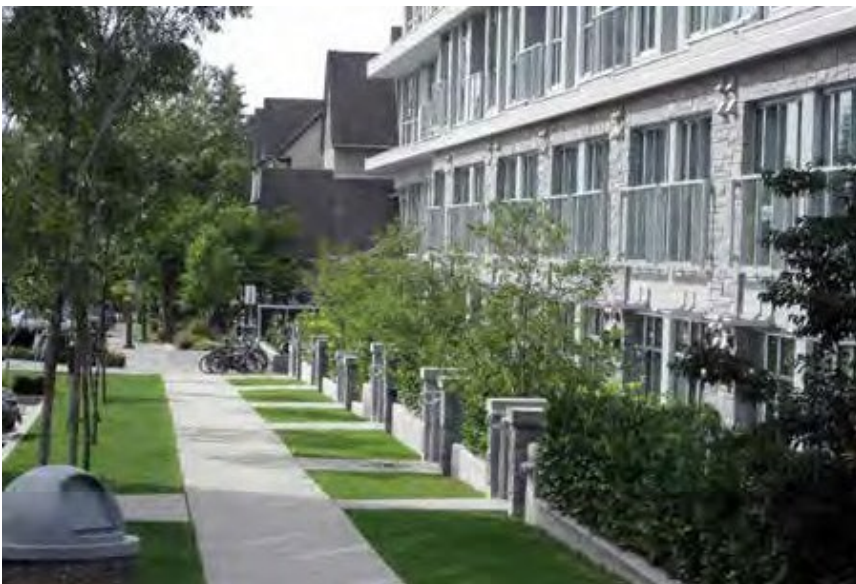
Individual Gates for Ground Floor Apartments
