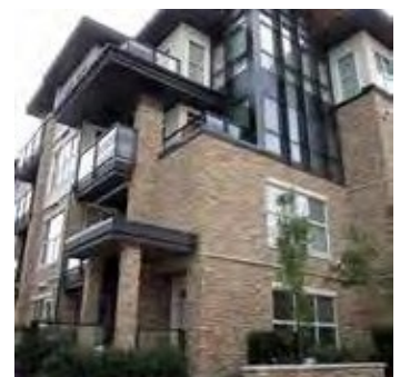
Outdoor Terraces Raised Above Street Grade
