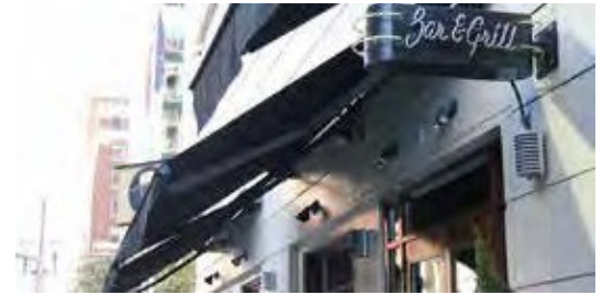
Weather Protection in Retail Area
