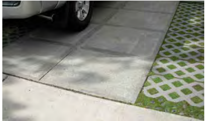
Cast-in-place concrete and permeable unit pavers
